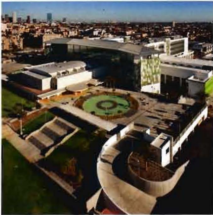
The two main buildings are separated by a 30-ft difference in grade, eased by incorporating a terraced outdoor amphitheater.
