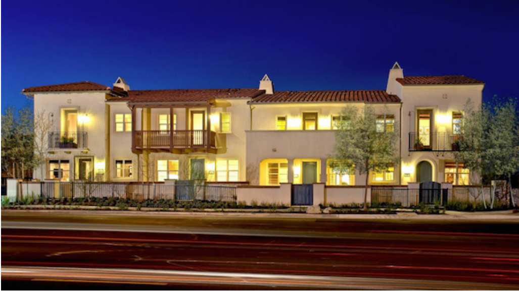
Each townhome has a private entry, private open space, and balcony.
